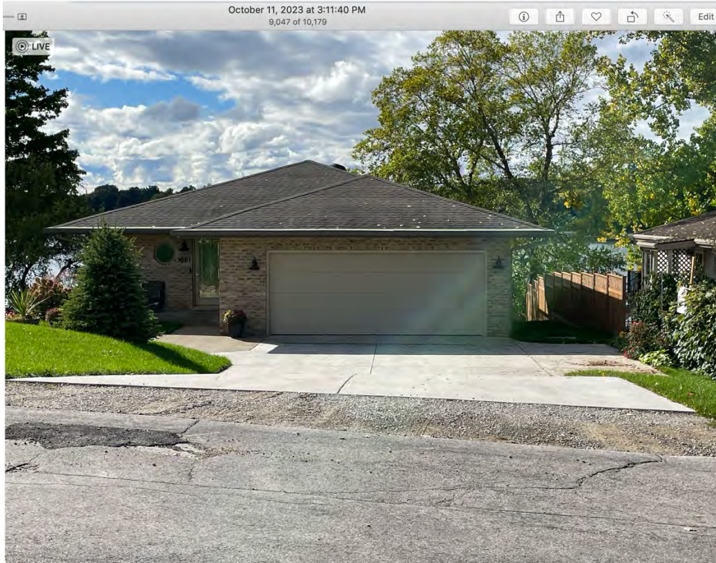
New Concrete: Note solid concrete from Apron to garage, driveway width now approx. 20ft, new south parking area, expanded north concrete in side yard adjacent to 1669 Lake Drive
