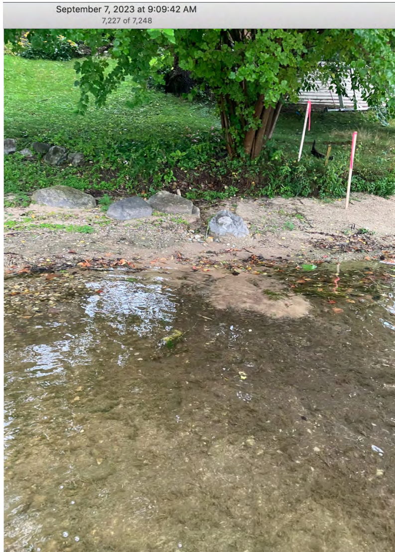
Sediment push into Silver Lake from September 2023 storm. This washout occurred after the storm system was 'completed'
