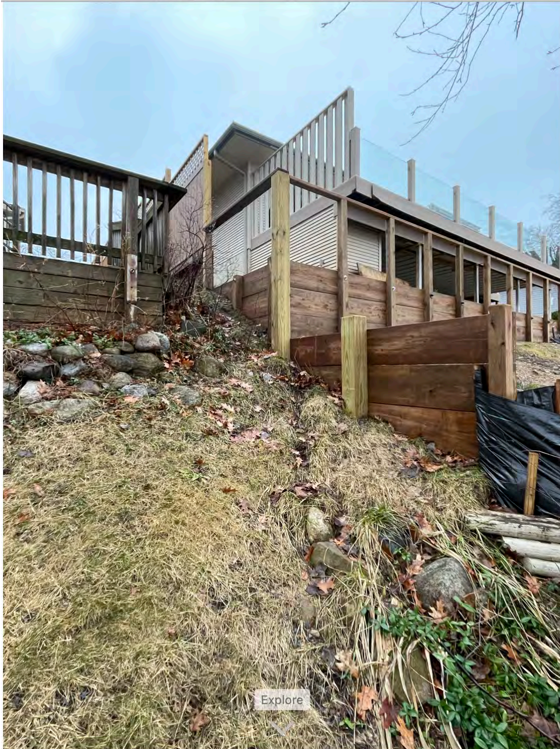
Water path from the corner of the lower drain. Erosion grid at 1669 Lake Drive is exposed in the foreground
