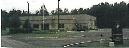
Station 1 843 Industrial Circle, East Bay Township
