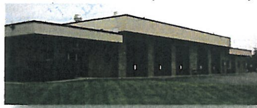
Station 11 3000 Albany, Garfield Township
