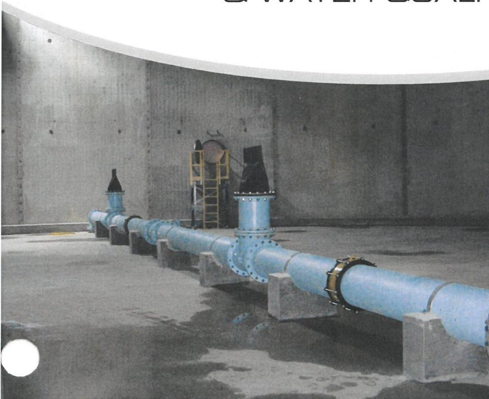
► In response to specific water quality design requirements, various mixing systems are available, ranging from separated piping, to flow-based systems, to mechanical mixing equipment.
