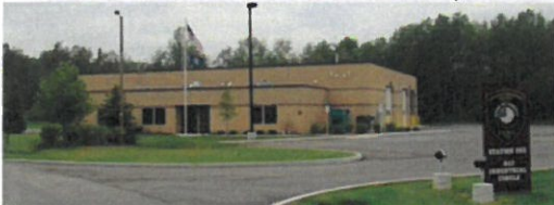
Station 1 843 Industrial Circle, East Bay Township
