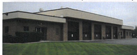
Station 11 3000 Albany, Garfield Township
