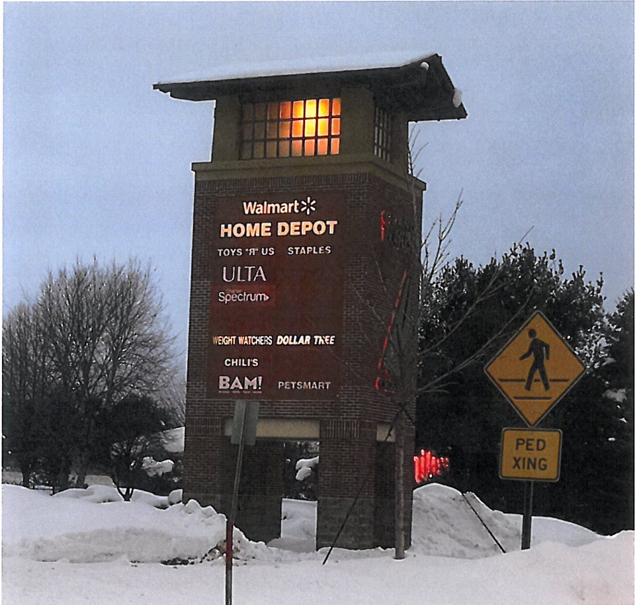
Grand Traverse Crossing freestanding sign structure with tenant panels
